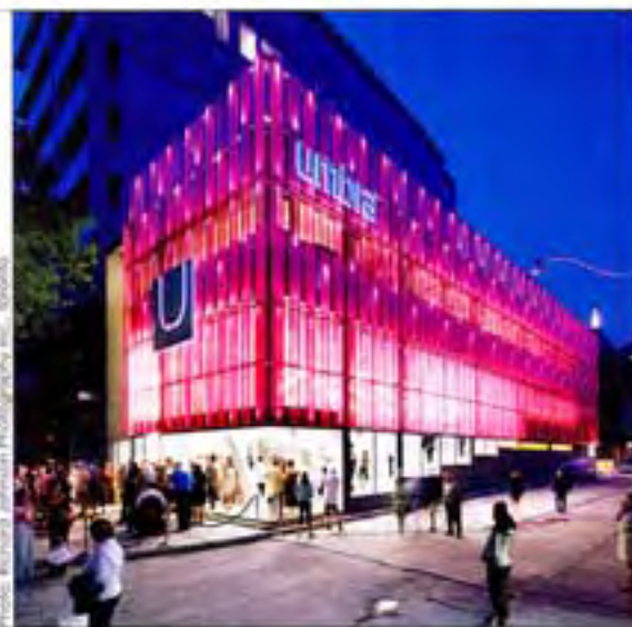
The exterior of Umbra's new Toronto store is surrounded by pink louvers that filter light in the day and glow at night.
